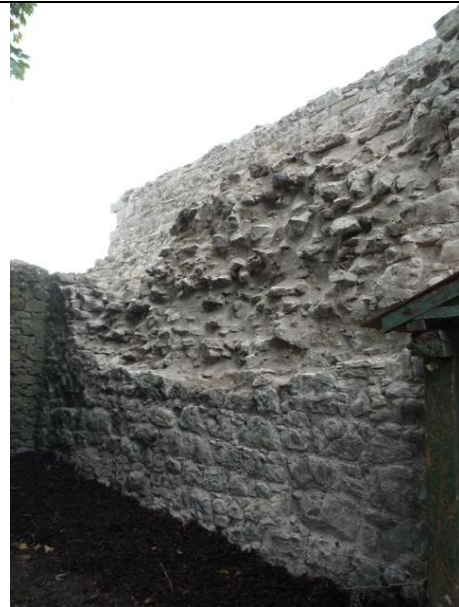
Fig.20: After - Consolidation of exposed core following removal of plantlife.
