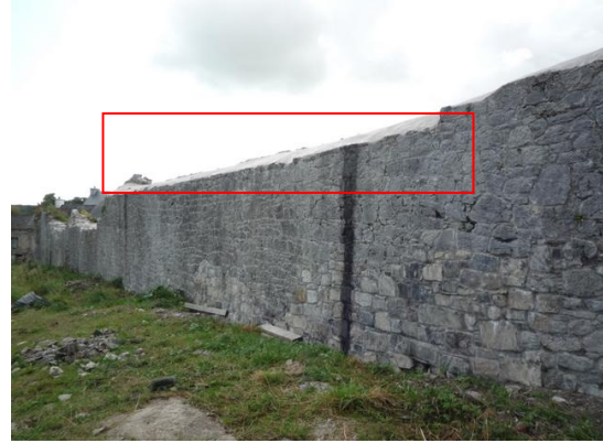
Fig.34: After - Section D following re-flaunching and removal of plantlife.
