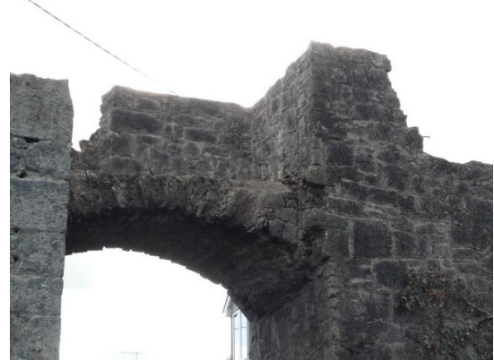
Fig.32: After - Wallwalk following removal of plantlife and flaunching of skyward surfaces.
