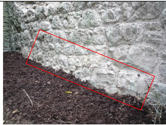
Fig.18: After - Patch repair of base stones to Section A.
