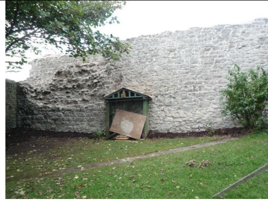
Fig.16: After - aspect taken following removal of the plantlife and consolidation of the wall.
