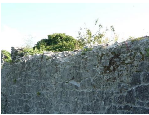
Fig.35: Before - Wall head prior to works.
