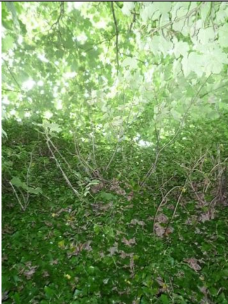
Fig.19: Exposed core concealed by heavy overgrowth.
