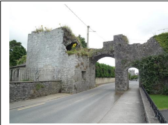
Fig.27: Before - North Gate and tower prior to conservation.
