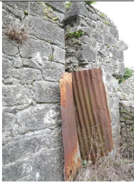
Fig.6: Breach in Section F of the Town Wall. Note that this has been temporarily blocked with a sheet of tin.
