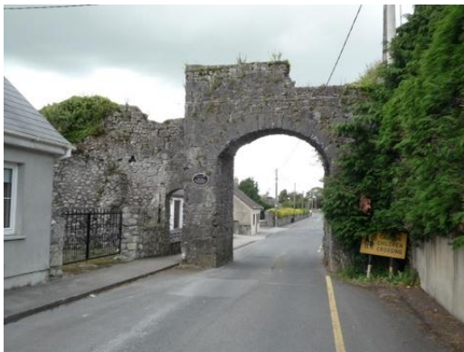
Fig.25: Before - North Gate prior to conservation works.
