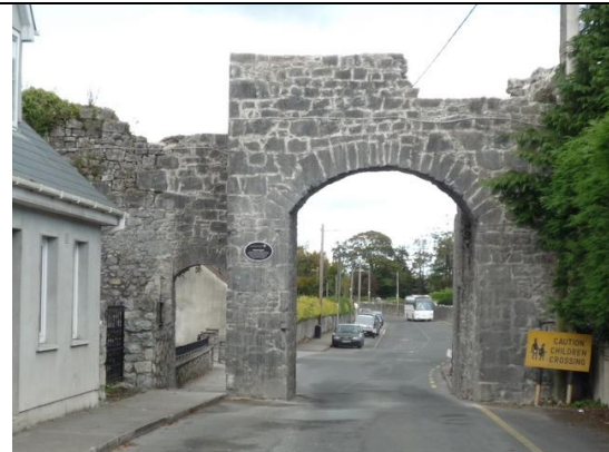
Fig.26: After - North Gate following removal of plantlife and re-pointing of elevation.
