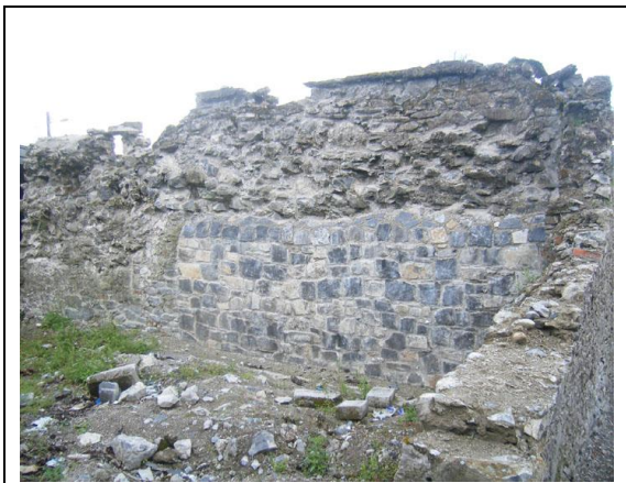
Fig.45: Section of wall to the east of Watergate.
