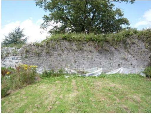
Fig.21: Before - Section B prior to conservation works.
