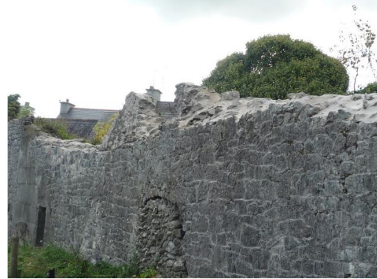
Fig.36: After - Consolidation of the wall head.
