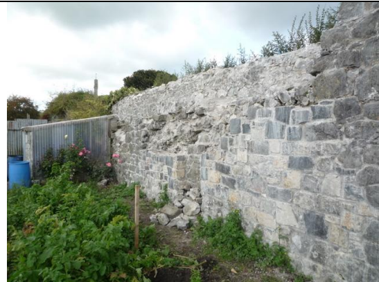
Fig.24: After - Section of wall following consolidation and removal of plantlife.
