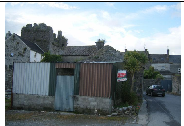
Fig.46: Lean-to structure at Watergate.
