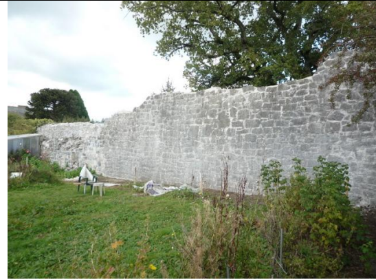
Fig.22: After - Section B following removal of plantlife and re-pointing of masonry.
