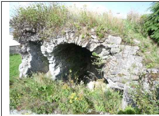
Fig.3: Significant plantlife to the skyward surfaces of the North Gate and tower.
