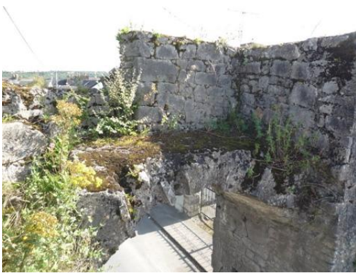
Fig.31: Before - Wallwalk and parapet over archway prior to conservation.
